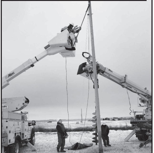
Black Hills Electric's Crew Foreman Dean Whitney and journeymen linemen Beau Bradeen, Ken Parker and Corey Scott replace poles near Red Shirt, S.D.
